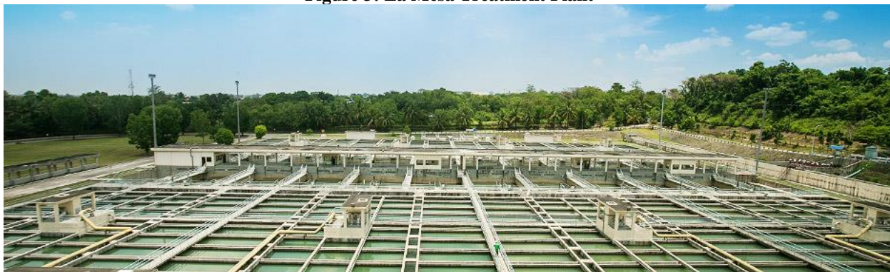
Figure 3: La Mesa Treatment Plant
